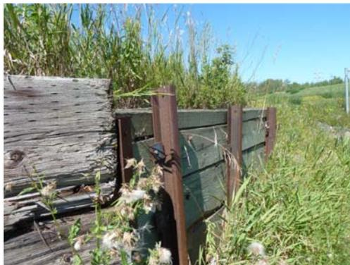
NW wingwall. Note crack in top plank.
